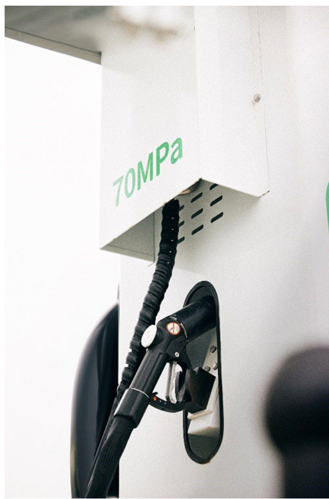
Hydrogen refuelling station for passenger cars (70 MPa) and heavy-duty vehicles (35 MPa).
