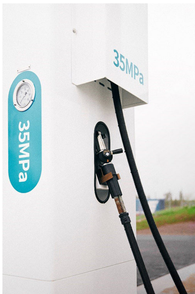
Hydrogen refuelling station for passenger cars (70 MPa) and heavy-duty vehicles (35 MPa).
