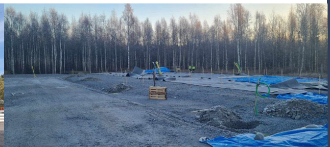
Groundwork from Piteå
